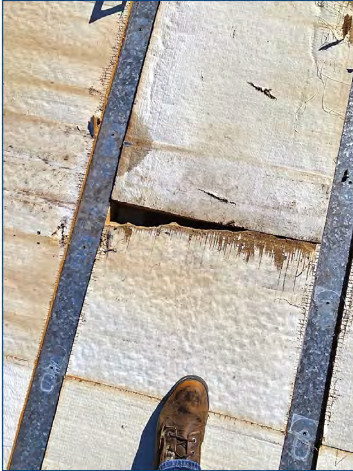
Figure 10 – Existing substrate after removal of metal roof at Tampa Airport.
